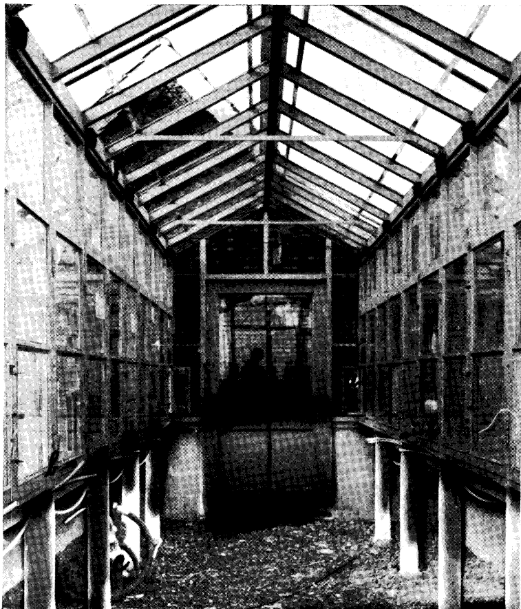
Fig. 2. — Central aisle in pollen-house. Compartments on both sides for pollen forcing. — a. Two panes opened to permit insertion and removal of catkin-bearing twigs (cf. fig. 3). — b. Plastic tubings, through which water containers can be filled or emptied without opening compartments. — c. Vacuum cleaner used for collecting (sucking up) pollen.
